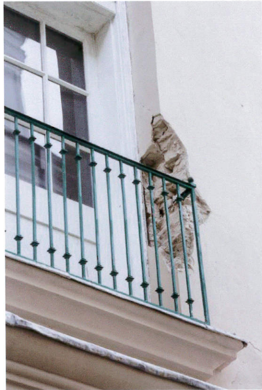
E3A1999 - Exterior: detail of second-floor balcony along Pere Antoine Alley
