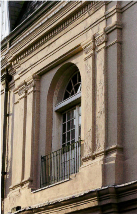
E3A1963 – Exterior: detail of second-floor wall section along St. Ann Street
