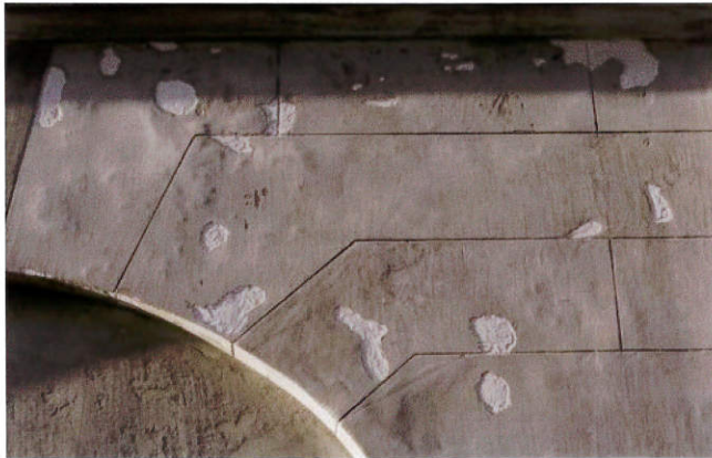
E3A1975 - Exterior: detail of first-floor wall section along Pirates Alley
