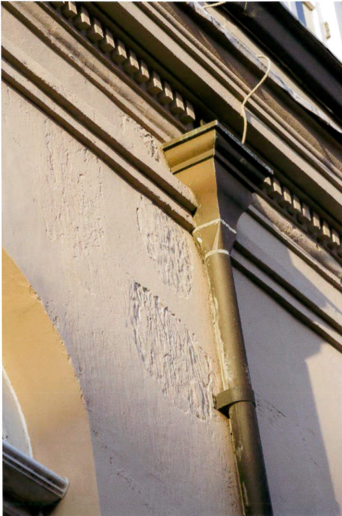
E3A1950 - Exterior: detail of second-floor wall section seen in photo E3A1967
