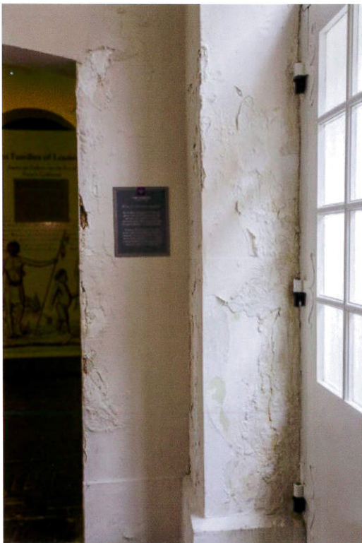
E3A2028 - Interior: detail of lower wall section seen in photograph E3A2027
