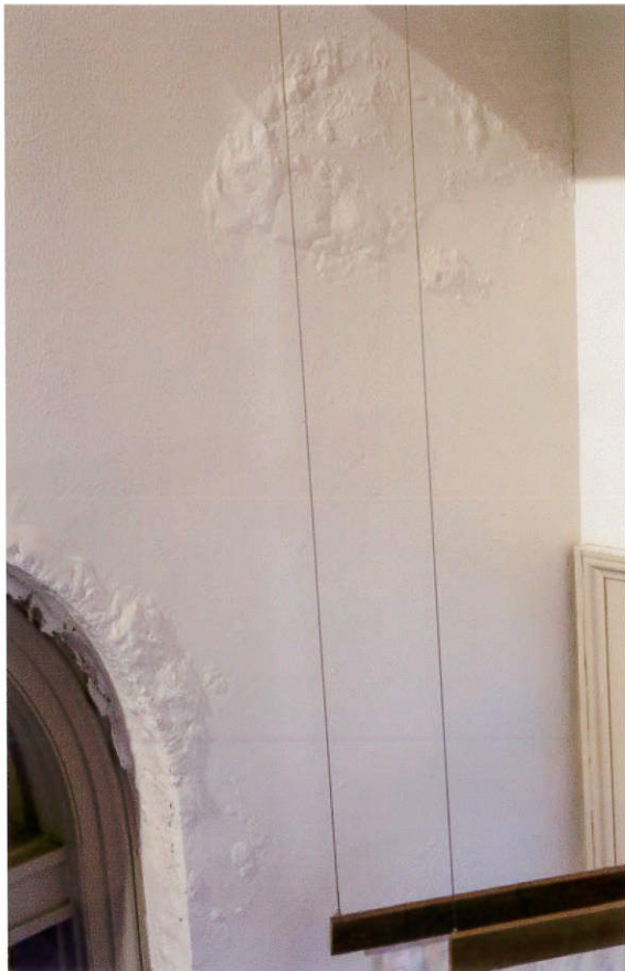
E3A2049 - Interior: detail of wall area seen in photo E3A2048
