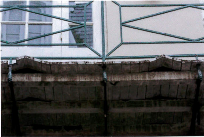
E3A1979 - Inner courtyard: detail of underside of balcony
