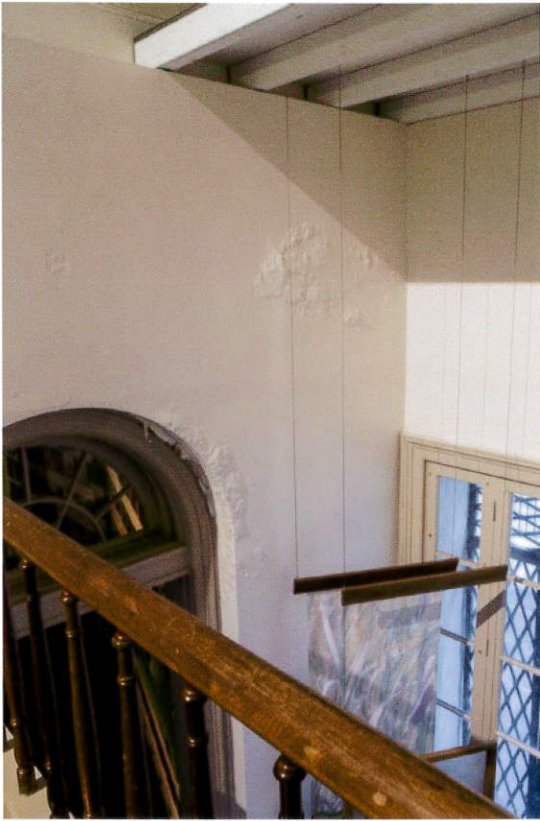
E3A2048 - Interior: view of wall area from main staircase's second-floor landing
