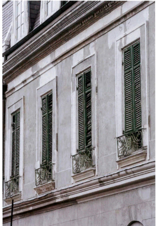
E3A2032 - Exterior: second floor shutters along St. Peter Street
