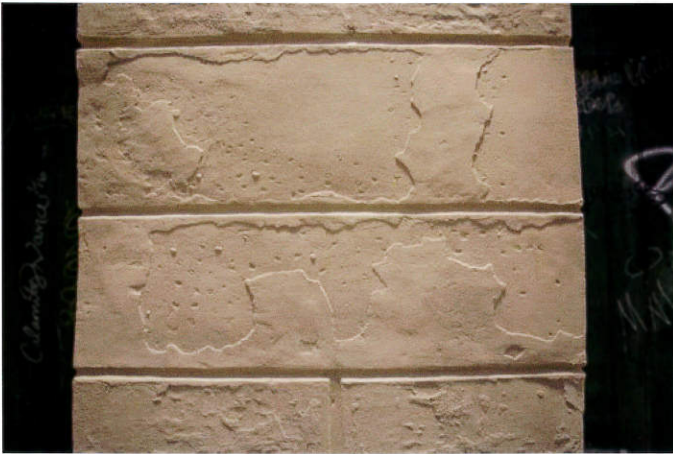
E3A1934 - Exterior: detail of wall section seen in photo E3A1933
